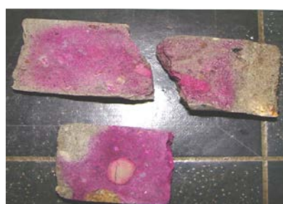
Figure 10. Pieces of Concrete A; visible layer into concrete with an alkaline pH, carbonized 1-3 cm in thickness.
