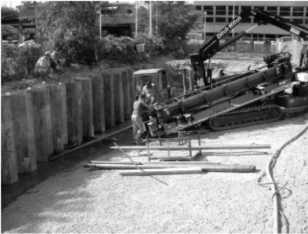
Fig. 35. Bologna tunnels: directional drilling in progress to install grouting tubes
