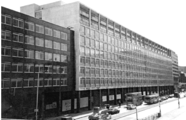
Fig. 44. Elizabeth House: detailed settlement monitoring during and after construction of Jubilee Line Extension
