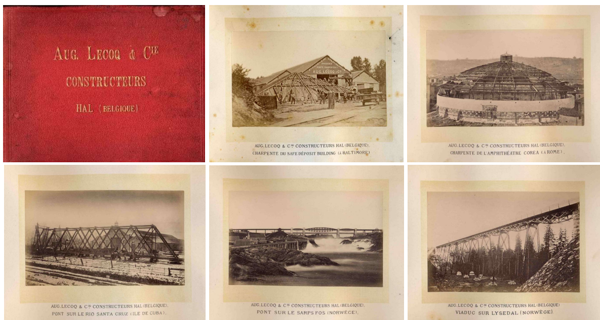
Figure 2: Trade catalogue Aug. Lecoq & Cie. Constructeurs Hal (Belgique) (c1880) depicting the roof truss of a safe deposit in Baltimore, the Corea Amphitheatre in Rome, a bridge over river Santa Cruz in Cuba, the Sarpsfos twin bridge and the Lysedal viaduct in Norway © het MOT, Grimbergen
