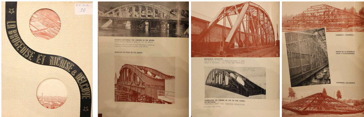
Figure 6: Trade catalogue La brugeoise et Nicaise & Delcuve (c1937) depicting the photos of the construction of the Vierendeel railway bridge Val Benoît in Liège (1935), a bridge in Argentina - a Vierendeel railway bridge for Congo (Bas-Congo au Katanga), roof trusses and the windscreen for the Alexandria station in Egypt © City Archive Bruges
