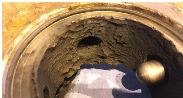
Fig. 1. Photo of corrosion defect of a tool flange.
