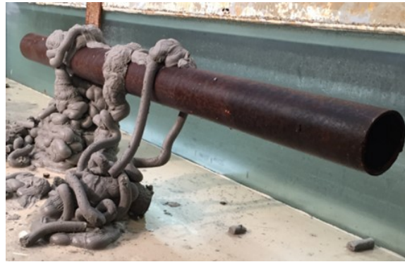
Figure 30 - Un-controlled Buoycrete application around steel pipe [11]
