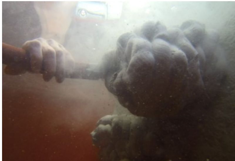
Figure 4 Application of a thick Buoycrete layer at a vertical concrete surface [41]
