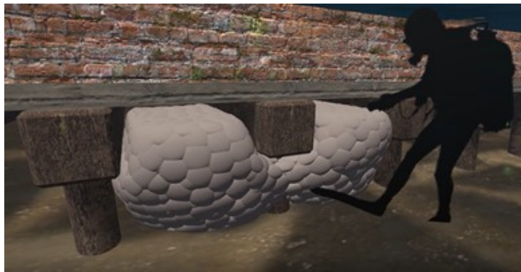
Figure 1: the underwater application of buoycrete in a membrane mould for the restoration of key walls
