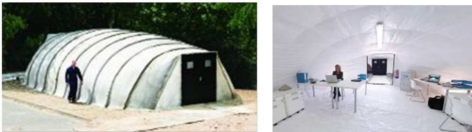
Figure 11 Concrete Canvas Shelter [16] Figure 12 Internal view of shelter [16]
