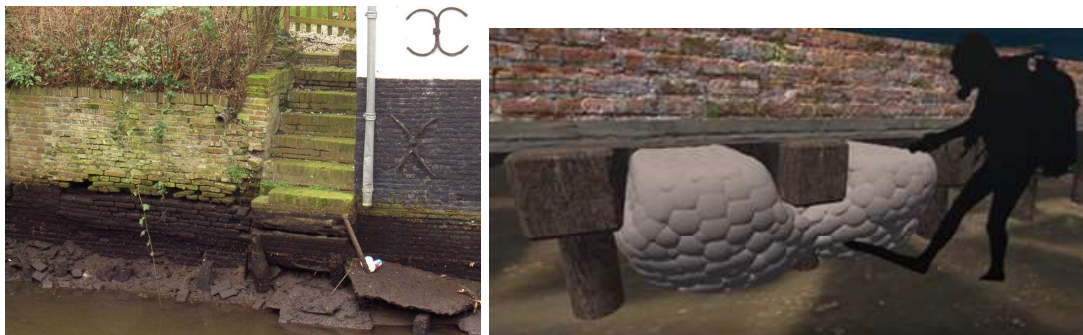
Figure 31 – Old key-wall Figure 32 – Restauration of key-wall with inflatable mould
