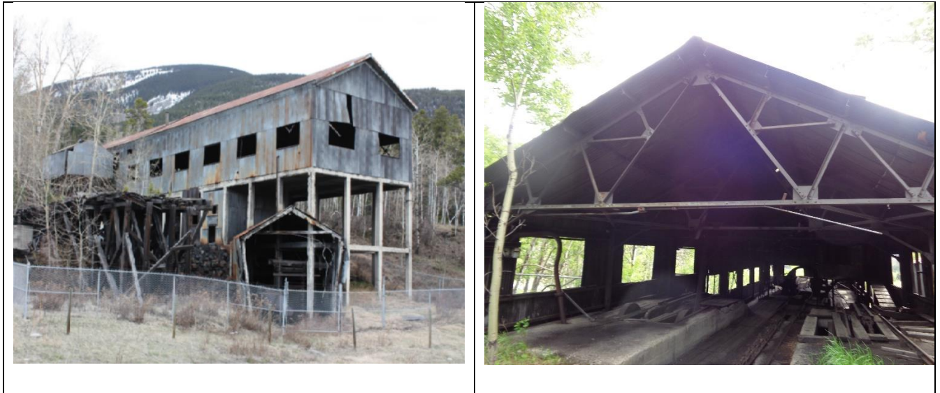
Figure 1: Overall view of Greenhill mine tippie structure and its roof trusses
