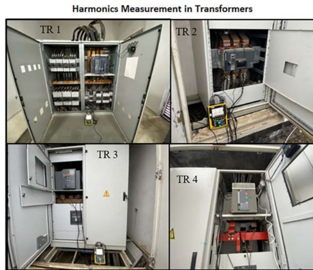
Figure 2: Transformer modular cells low voltage panel harmonic measurements
