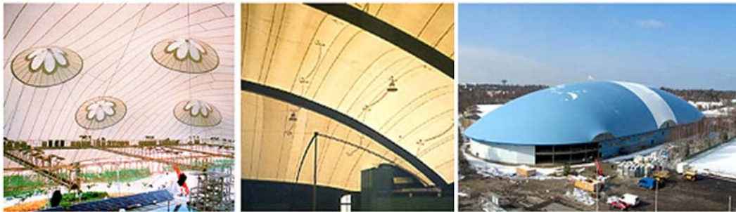
Figure 28: Schlaich & Bergermann, 1998: National Swimming Pool, Kuala Lumpur. The parallel membrane strips running towards the edge reflect the distributed stress caused by wind suction. The radial pattern of the high points reflects the concentration of loads due to snow. Figure 29: The layout of the patterns minimizes the waste but the result is messy and confusing. Figure 30: Matti Orpana, Tensotech: 14.300 m 2 inflatable football field in only one panel to avoid joining on site.
