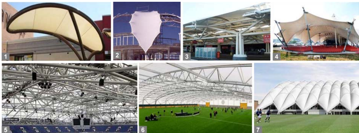
Figures 1, 2: Different approaches to design the edges of a membrane. Figures 3, 4: Different approaches to design the support structure. Figures 1, 3, 5, 6, 7: Steel structures clad with membranes. Figures 2, 4: Membrane structures.
