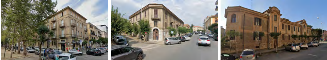
Figure 2: Some pictures of the studied masonry structures.
