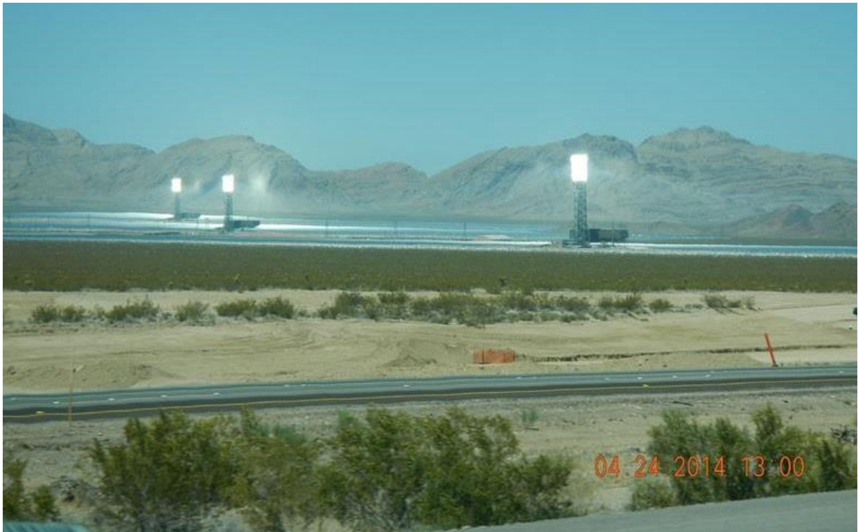
Figure 13. Photograph of illuminated receivers at Units 1, 2 and 3 while heading northbound along I-15.
