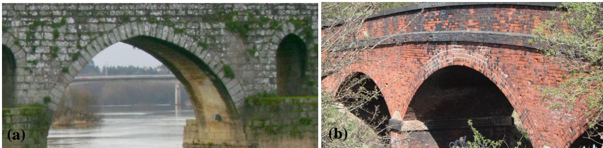
Figure 1: (a) Roman stone-bridge over the Limia river (Portugal) and (b) Brick Rail bridge, Stapleford (UK).
